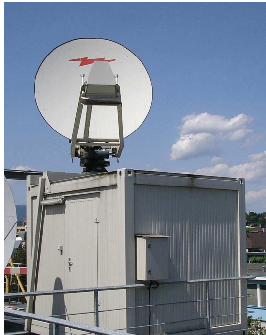
Fig.3: Graz Ground Station
